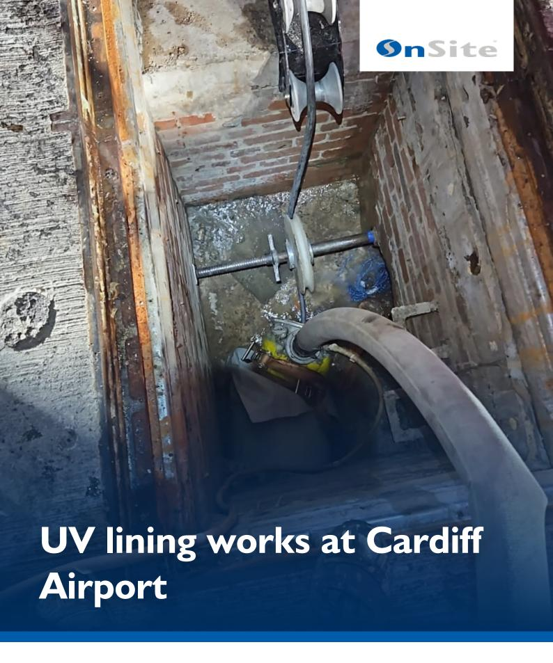
OnSite Rail was contracted by Forestry, Rail & Civils Ltd (FRC) to complete UV lining works on a pipe underneath Cardiff Airport.
