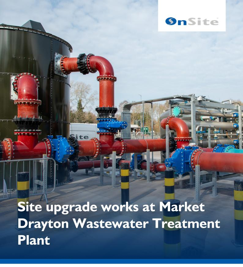
OnSite was contracted by Severn Trent Water (STW) to carry out site upgrade works at Market Drayton Wastewater Treatment Plant as part of a newly established Batch X Direct Delivery Model. This included the installation of a new chemical dosing plant and the construction of a tertiary solids removal (TSR) system and associated equipment.
