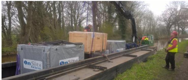
OnSite floating their portable UV Lining equipment to site using a canal barge. This method of delivery saved the client over £25k alone on the cost of matting that had been specified for access across third party
