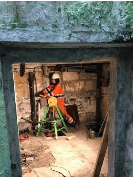
Access to upstream manhole inside the vault
