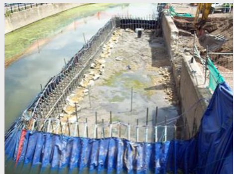
Outfall construction at the Olympic site
