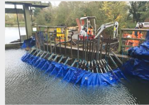
Outfall construction River Great Ouse
